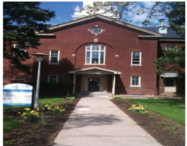
Main Entrance to LVR Offices, located in rear of building
